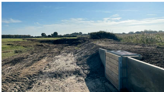
The New Sluice
