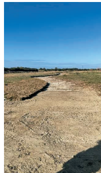
New low point winding from the lagoon to the solar pump location
