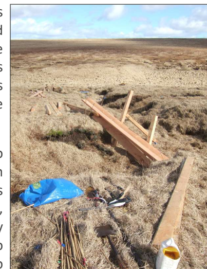
Timber for blocking gullies
