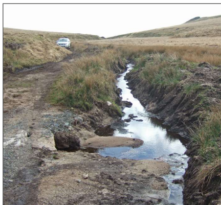
Newly dug drainage channel
