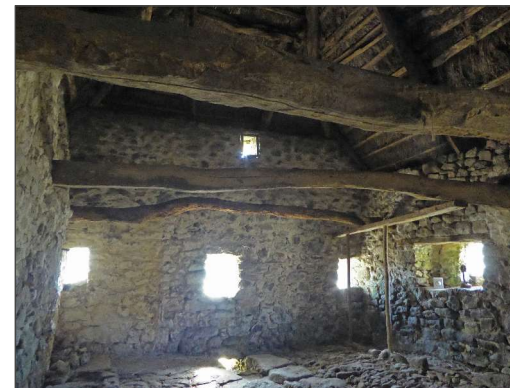
The shippon with 'owl hole' and livestock tethering posts
