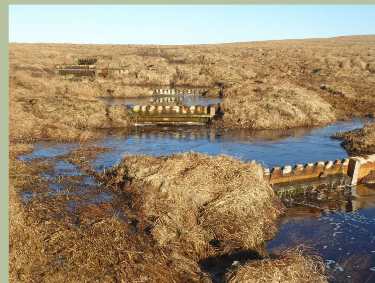
Series of leaky wooden blocks in Vergyland Combe
