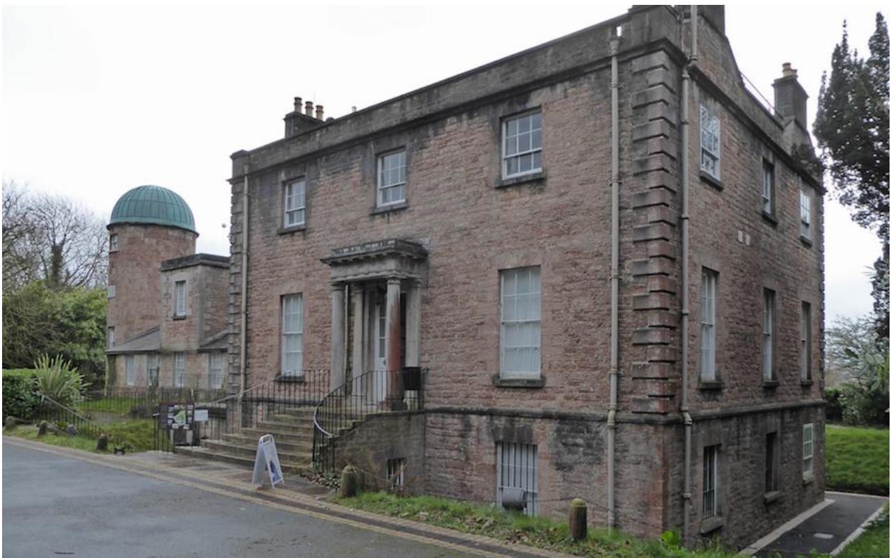
The front of the Observatory today, with the original 1790 Georgian building to right, and the later editions (going to left) of the Sector Tower (to house King George III's instruments from his Kew Observatory gifted by Queen Victoria), built over the Transit Room containing the Transit Instrument, then the Meridian Room with the Mural Circle, and finally the 1827 Tower.
