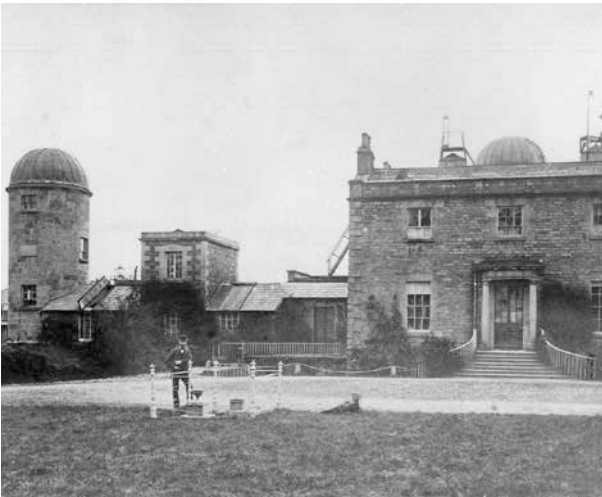
Historic image of the Observatory from about 1883, taken from the North Lawn with the meteorological enclosure in the foreground, with the 4 th Director Dreyer beside it. On the roof can be seen the Robinson cup anemometer. To left is the East Tower with its 1827 Dome, built following a bequest from Archbishop Beresford and containing the Grubb 15-inch reflector telescope with a then novel lever support system for the mirror.
